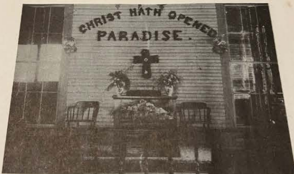
CHANCEL of the FIRST METHODIST CHURCH OF GENEVA, FLORIDA
